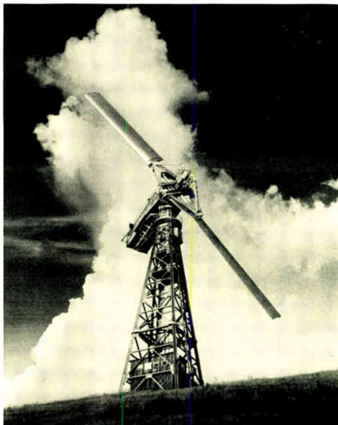
... The windmills of Holland and the American farm-yard have captured much useful power from the winds, but it is insignificant compared to our needs. On Grandpa's Knob on a Vermont mountain top is this wind-driven power plant, delivering at full load 1000 kw. (Photo courtesy S. Morgan Smith Company.)
