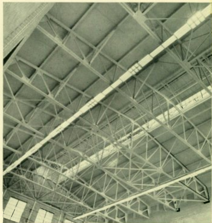
The illumination needs of a power-house turbine room are served by this unique custom-built lighting installation. In these two lines of light, 40-watt fluorescent lamps are used in conjunction with 500-watt filament lamps to provide light of a pleasing color. Despite the high mounting height of 60 feet, the average illumination is 22 footcandles.
