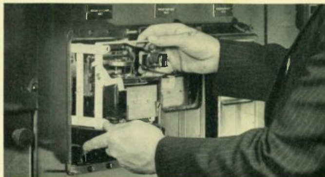
The ease with which the relays are removed from the new Flexitest case is demonstrated in the photograph above while the manner in which the relays are tested by integral switches is shown below.
