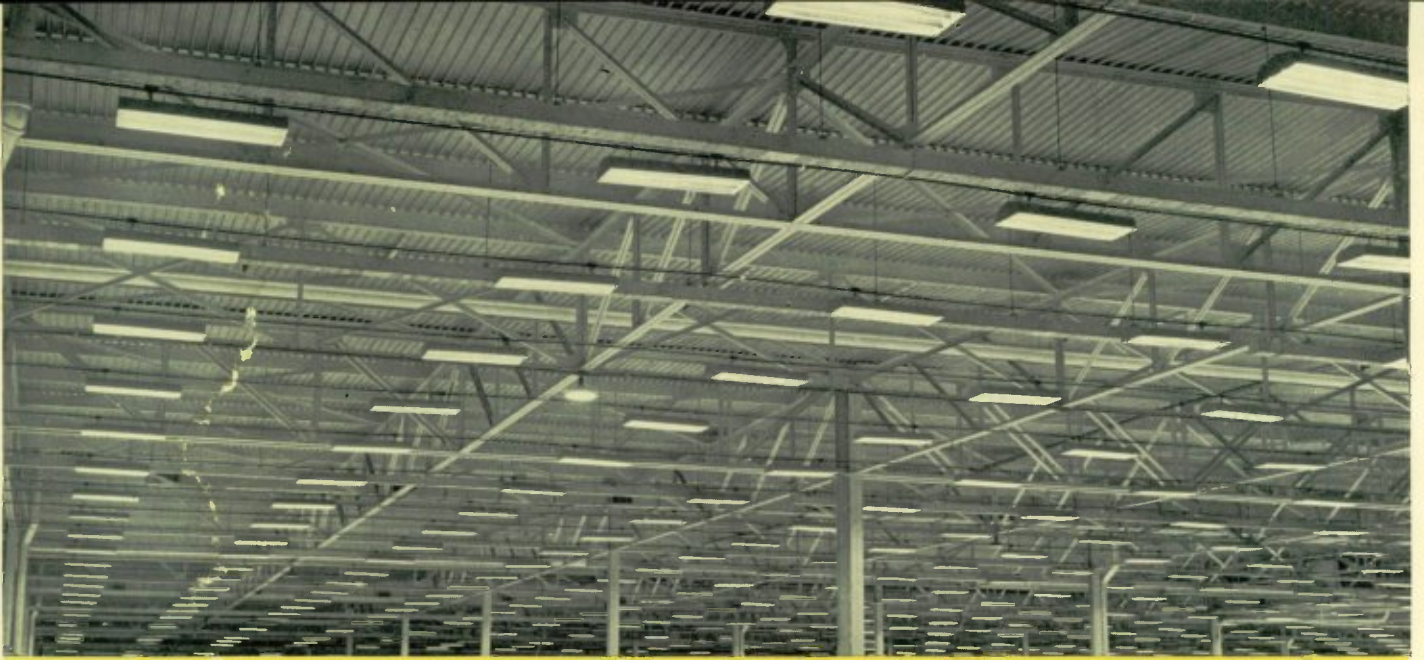
Fourteen miles of fluorescent tubes light the prefabrication and manufacturing areas in the Kansas City plant of North American Aviation Inc. Here well-diffused light eliminates the need for supplementary lighting for most of the underneath work on the Mitchell bombers. Adequate intensities are provided for highly precise machining operations and small-tool production without specular glare and minimized direct glare.
