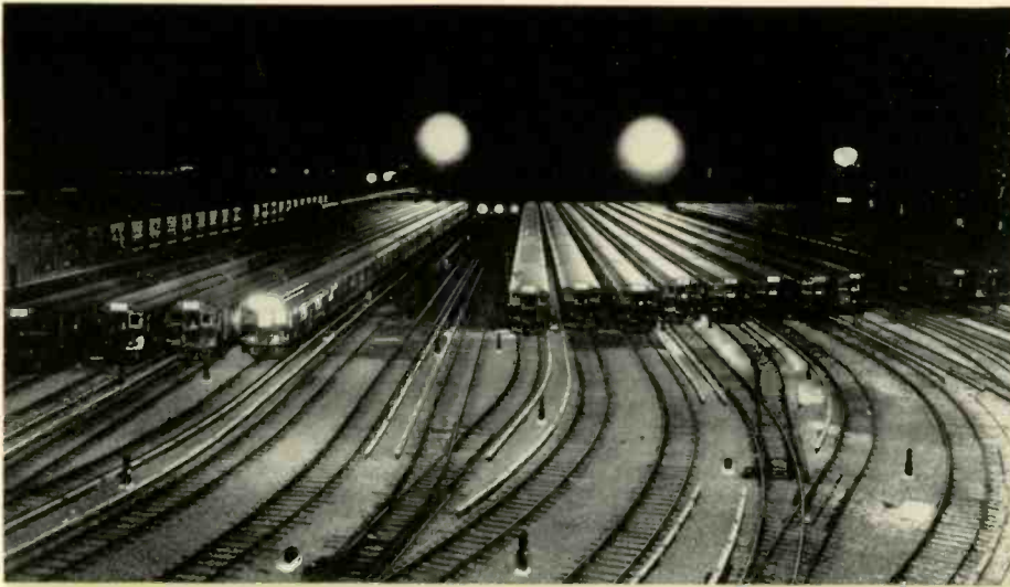
Taken from the "Illumination—Fundamentals and Application" training film, this picture gives an example of the results of adequate floodlighting within a train yard.
