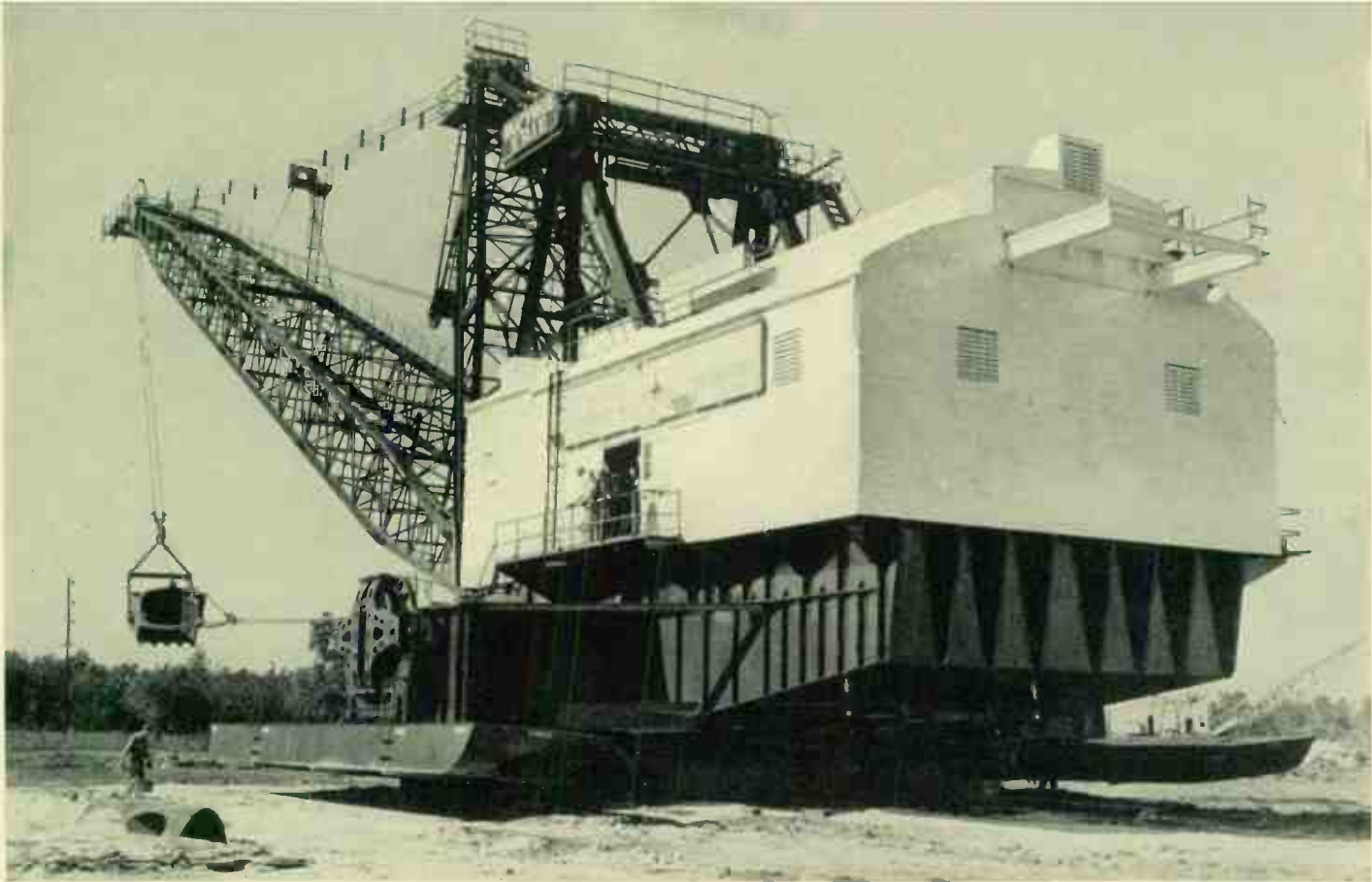
Phosphate ore is mined with draglines like this latest walking type with a 215-foot boom and a bucket capacity of about 25 tons.
