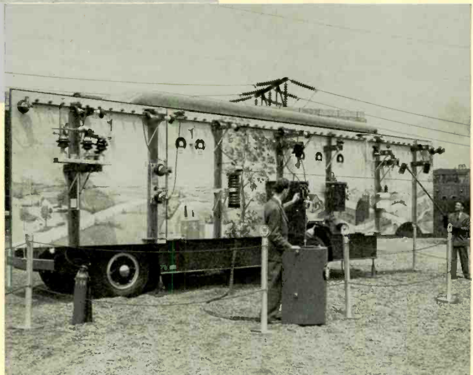
The principles and basic equipments of electric-power distribution and its protection are visibly displayed by a distribution system on wheels. A surge generator makes possible the demonstration of each type of protective apparatus.
