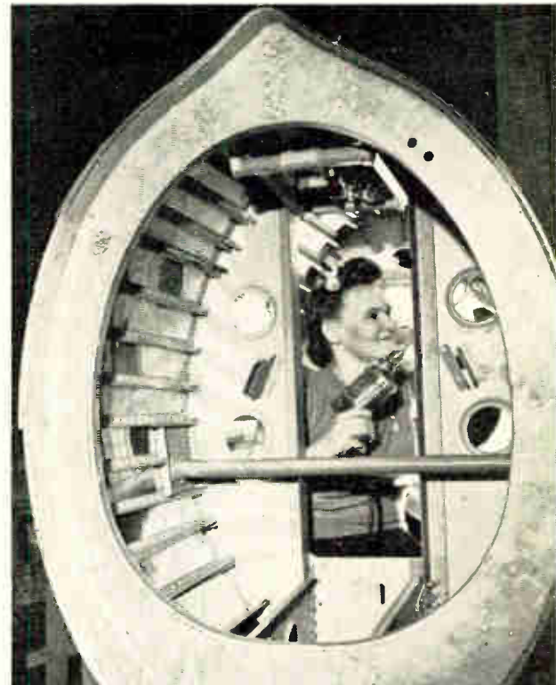
⚡ Standing by the bulkhead of a cone, Millie Moore does the necessary drilling before riveting the aluminum skin to the framework.
