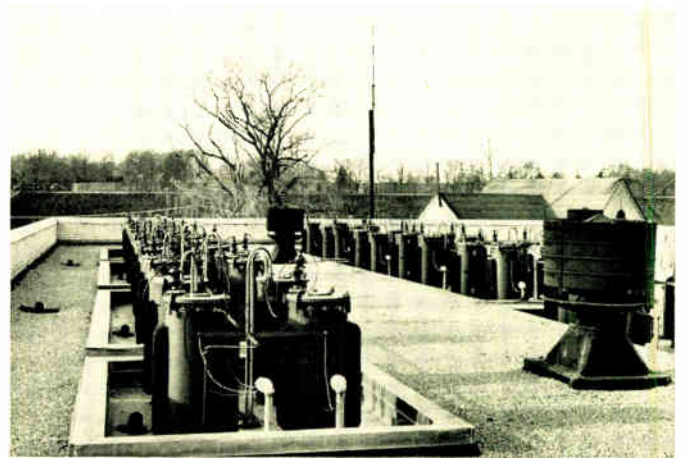
The fifty transformers that supply Belmont's ozone generators.
