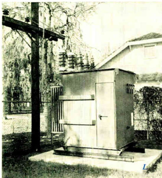
L (left)—A 1000-kva CSP power transformer for single feeders on a Texas utility company system. M (right)—A 4000-kva unit substation on a Pacific Coast utility system. High voltage: 69 kv. Low voltage: 12 kv.
