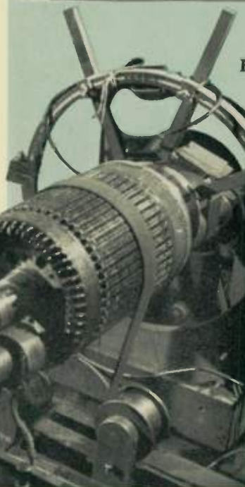
The second type of surge-comparison tester, possessing some additional features over the portable or table model, is shown here in service checking: (A) the stator insulation of a high-voltage generator, (B) a small-d-c armature, and (C) the stators of fractional-hp motors.
