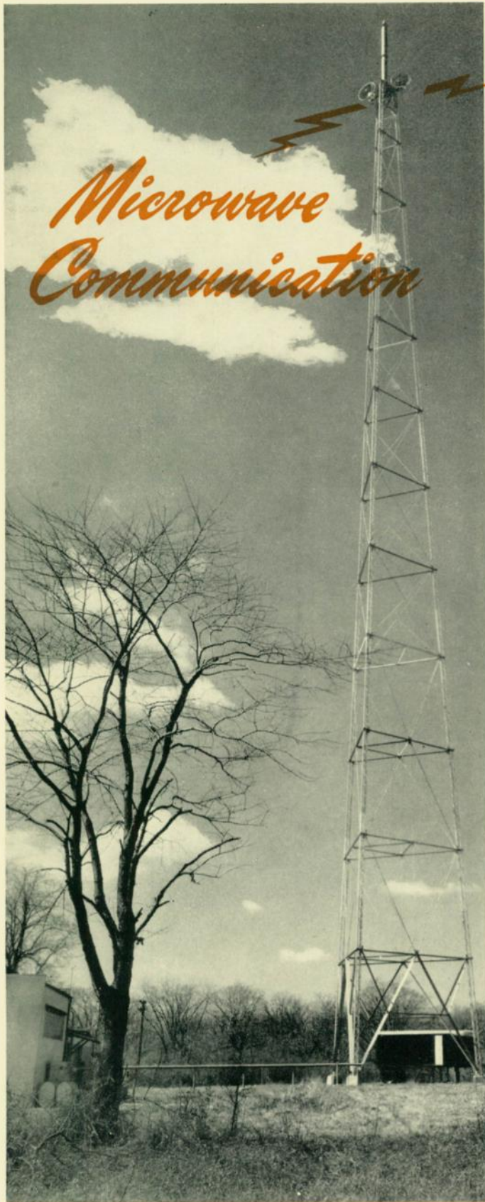
Microwave signals are relayed at this repeater station, which is a part of a complete system at Baltimore, Md.
