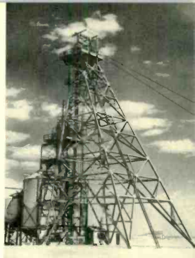
A typical headframe over a mine shaft, where ore is raised to the surface.
