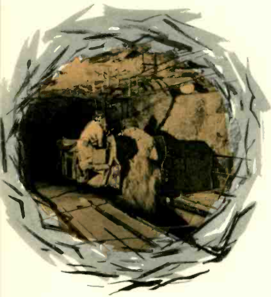
Shuttle car unloading into dumping pocket.
