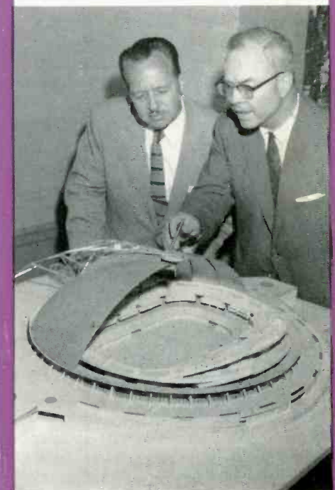
Model of Pittsburgh's civic auditorium, which will be capped with the world's largest movable dome—415 feet in diameter. At the touch of a single control button, six roof leaves will move at differential speeds to arrive at the open or closed position in the same time—2½ minutes! The leaves will move at predetermined, synchronized speeds, governed by speed and horsepower of each leaf's five electric drive motors and by individual reactor controls for each leaf.
