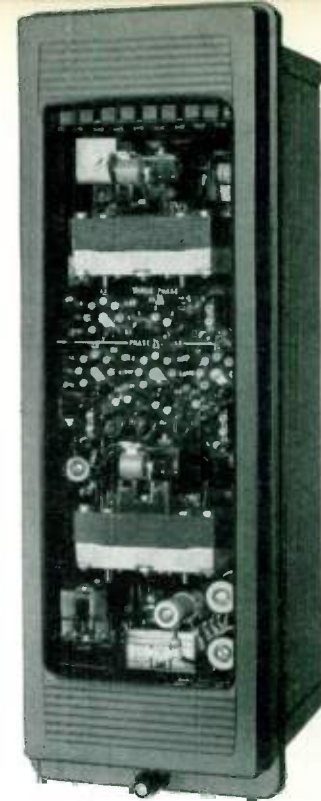
Fig. 5—Type KD compensator distance relay.
