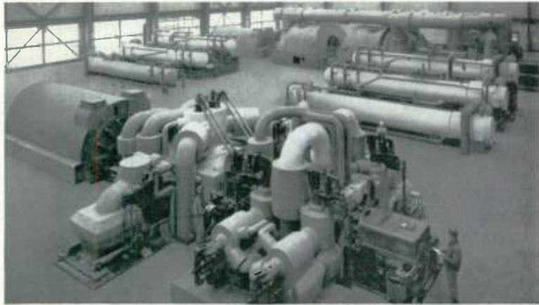
Photo 1 This 325-mw super-pressure steam turbine, now in operation at Philadelphia Electric's Eddystone station, has the highest steam conditions of any machine in service. The unit went into commercial operation in February 1960. It is nearing the end of a starting program during which pressures and temperatures were increased in steps.
