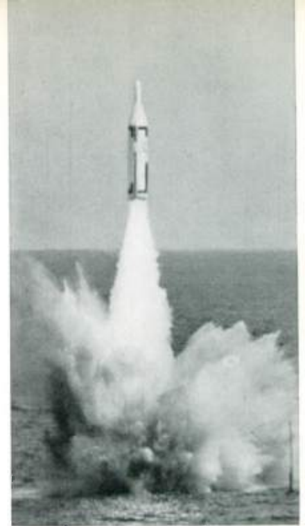
The Polaris , the solid fueled intermediate range missile, is shown after launching from a submerged submarine. The compressed-air launching system, developed by Westinghouse, is designed for either surface or underwater launching. Under a U.S. Navy contract, Westinghouse is building the launching and handling systems for a total of 14 missile submarines.
