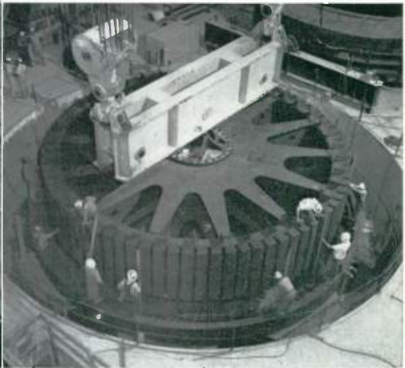
tric Project of Public Utility District No. 1 of Chelan County, Washington. (a) This aerial view looking upstream shows final-stage construction of the dam and powerhouse. (b) Unit 4 generator, shown during installation, is the fourth of seven 107 000-kva water-wheel generators being installed. The machines will operate at 90 rpm with a head of less than 100 feet.
