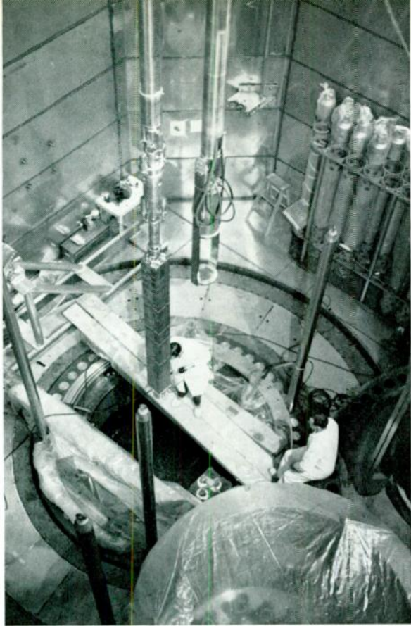
A fuel assembly being lowered into the nuclear reactor during the initial loading.
