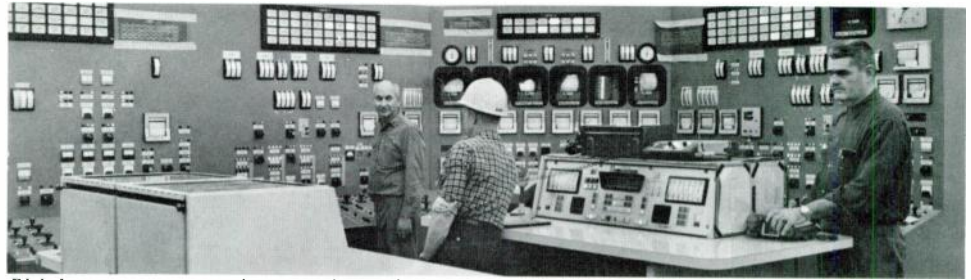
Digital computer system supervises a central generating station.
