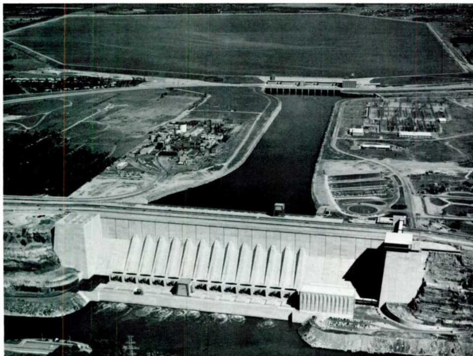
The 60,000 acre-foot capacity reservoir (background) of the Niagara Power Project permitted installation of an additional 240,000 kilowatts of capacity, bringing total project capacity to 2,190,000 kilowatts.
