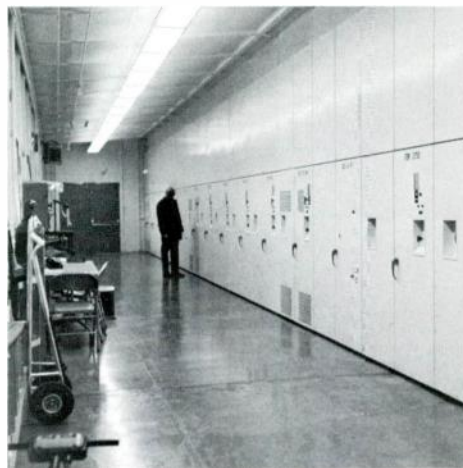
8—The first installation of the 34.5-kV metal-clad switchgear with an outdoor Sheltered-Aisle enclosure was at the East Pine Substation of Seattle City Light, Seattle, Washington (top.) Indoor view of this same installation (bottom) shows the wide aisle space provided for handling and servicing breakers.
