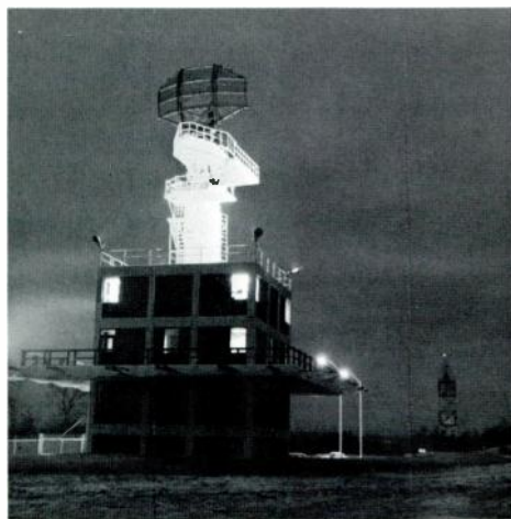
Control building in the radar antenna test complex has receiver mounts on its balcony and roof. The main mount extends 30 feet above roof level and provides ability to test very large antennas. In the background is the range's low-frequency transmitter tower.
