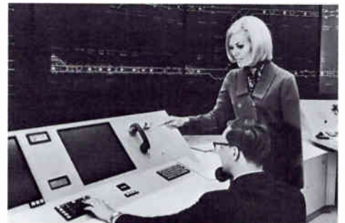
Train operations control center for Bay Area Rapid Transit includes a display board that depicts various functions of the 75-mile system. Tight automatic control of the trains will permit safe operation at speeds to 80 miles an hour and spacing as close as 90 seconds.
