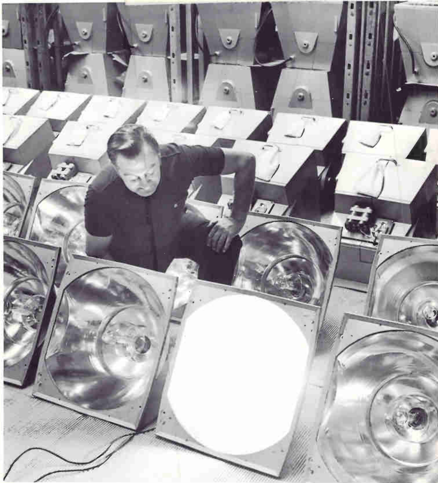
Maintenance-free floodlights for new Pittsburgh stadium. (Information on page 128.)
