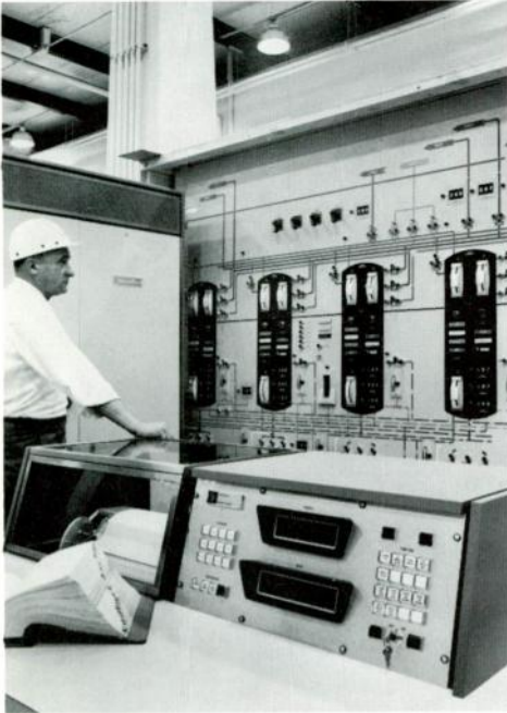
Operator's console is the user's main link with his process, so it should be specified for easy and effective communication to and from the process. Such "human engineering" techniques as color coding should be considered.
