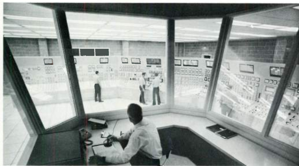
Instructors use this console to introduce simulated plant malfunctions into the program of the nuclear plant simulator. They observe the student's reactions in the control room.
