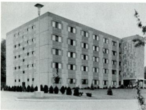
WATERBURY, Connecticut—Mall View Apartments, the Northeast's first Bison building, was completed in early 1972. It is a five-story 86-unit HUD turnkey housing development for the elderly. Using the Bison wall frame system, Blakeslee erected the basic structure of precast concrete components in just 7 weeks. Total time from groundbreaking to building dedication was 6 months.
