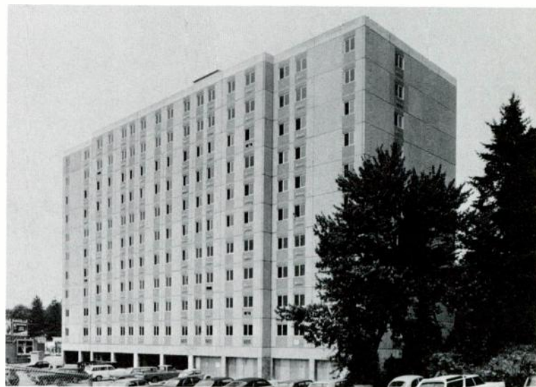
BRIDGEPORT, Connecticut—Park Towers, a 10-story 109-unit apartment building, provides semi-luxury housing for its occupants. Along with many other advantages, the building developer chose the Blakeslee precast building system because it permitted him to deal with just one major subcontractor for the manufacture and erection of the basic building shell.
