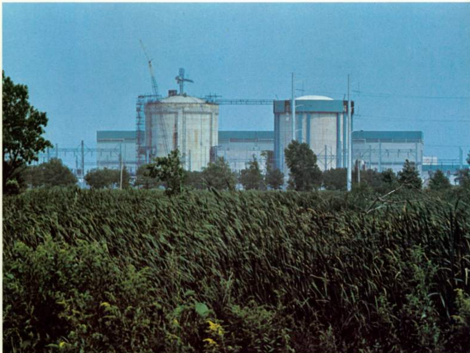
A Westinghouse nuclear reactor system rated at 1100 MW has gone into operation at Commonwealth Edison Company's Zion nuclear power station, Zion, Illinois. It is housed in the reinforced-concrete containment structure at right. A similar unit, in the structure at left, is scheduled for operation early this year.
