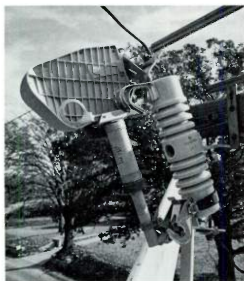
2—The fused distribution limiter employs a series combination of current-limiting fuse (larger diameter) and expulsion fuse (smaller diameter). The fuse combination is sized for direct replacement of the standard expulsion fuse in all Westinghouse loadbreak and nonloadbreak assemblies manufactured since 1962.
