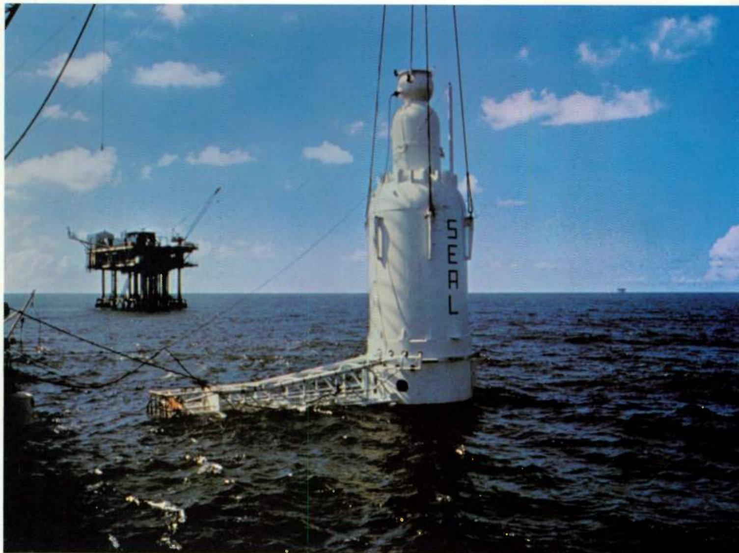
Part of a multiple-well production/manifold center for ocean-bottom oil and gas production is being lowered into the sea in this photograph. It is the center's work enclosure, and maintenance crews will be transferred to it when needed. For more information, see page 92.
