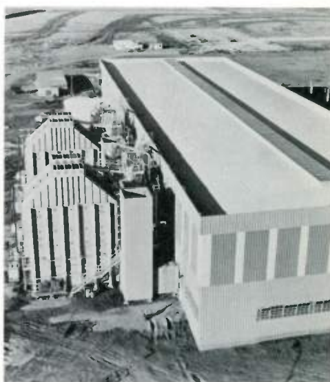
The PACE plant covers less than an acre and has a low profile, appearing more like a small industrial building than a conventional power plant. Its two heat-recovery steam generators, at left, produce steam for the steam turbine from the exhaust heat of the two gas turbines.
