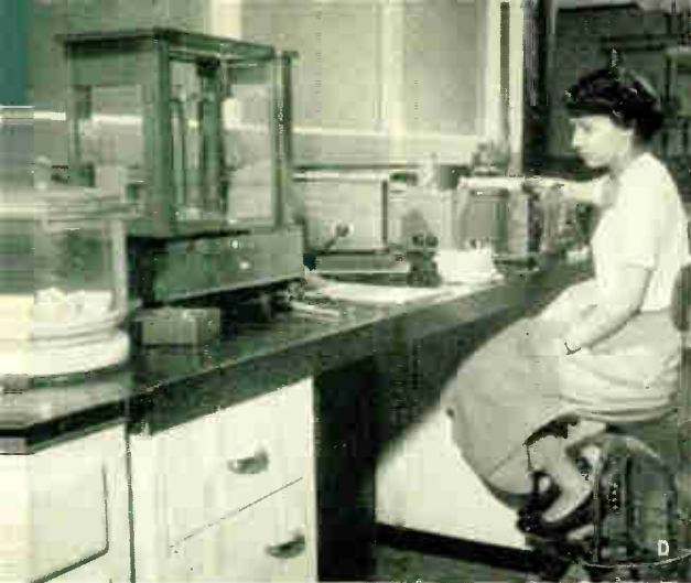
D —Tattle-tale grey concerns laundry-equipment designers. A reflectometer checks fabric whiteness.
