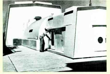
1150-KW BRUSHLESS EXCITER provides excitation power for 243-mva turbine generator at the Asheville Steam Electric Generating Plant of Carolina Power & Light Company.
