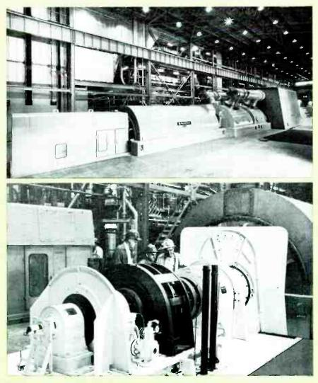
TURBINE GENERATOR UNIT THREE of West Penn Power Company's Mitchell Station is rated at 352 mva. The housing on the left end of the turbine generator contains the 1350-kw brushless excitation system. Brushless exciter system is shown with the housing removed (below). From left to right, major components are pilot exciter, ac exciter, fuse wheels, and diode wheel.
