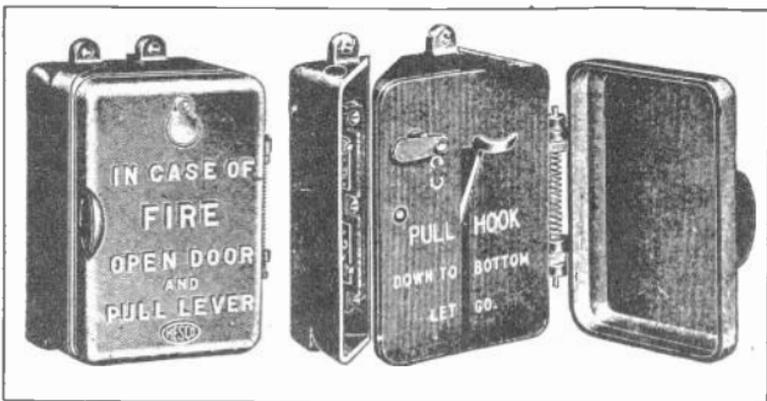
Fig. 11. Another type of fire alarm pull box which also sends code signals.
