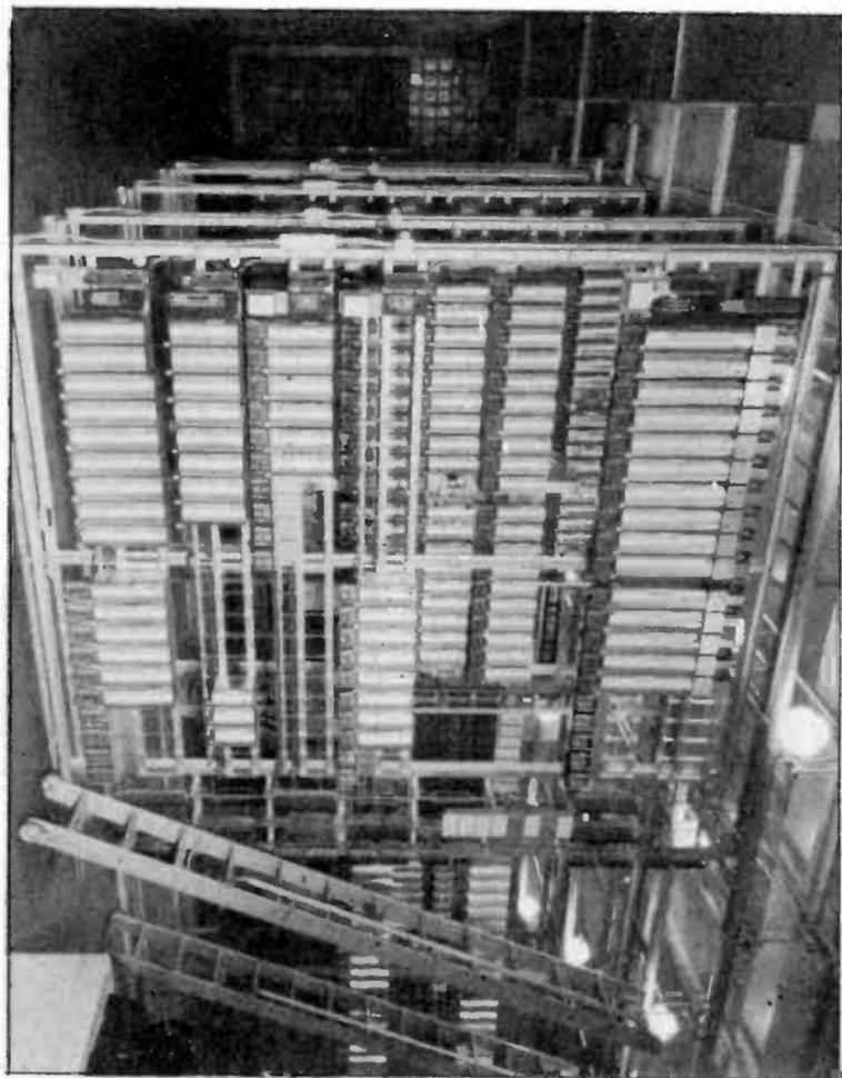
Strowger (Step-By-Step) Dial Telephone Switching equipment (Installed at Logansport, Indiana).
