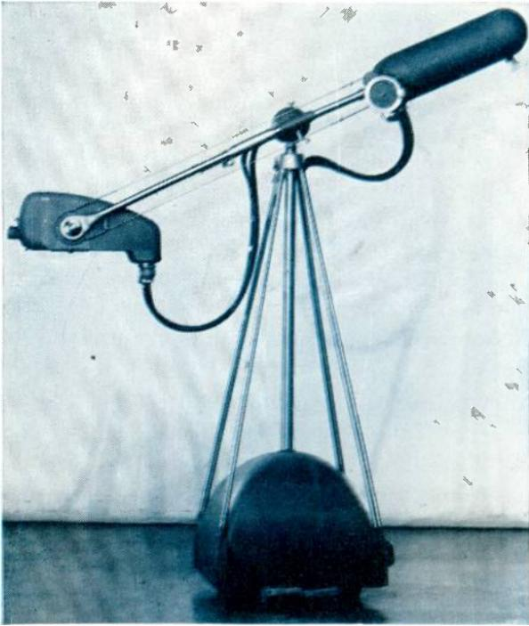
Fig. 18-15.—CBS color television camera mounted on a counterbalanced boom.
