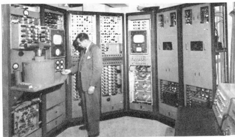
*Fig. 18-1.—General view of equipment which includes studio control units of the new RCA all-electronic high definition compatible color television system as installed at the NBC station WNBW, Washington, D. C.*
