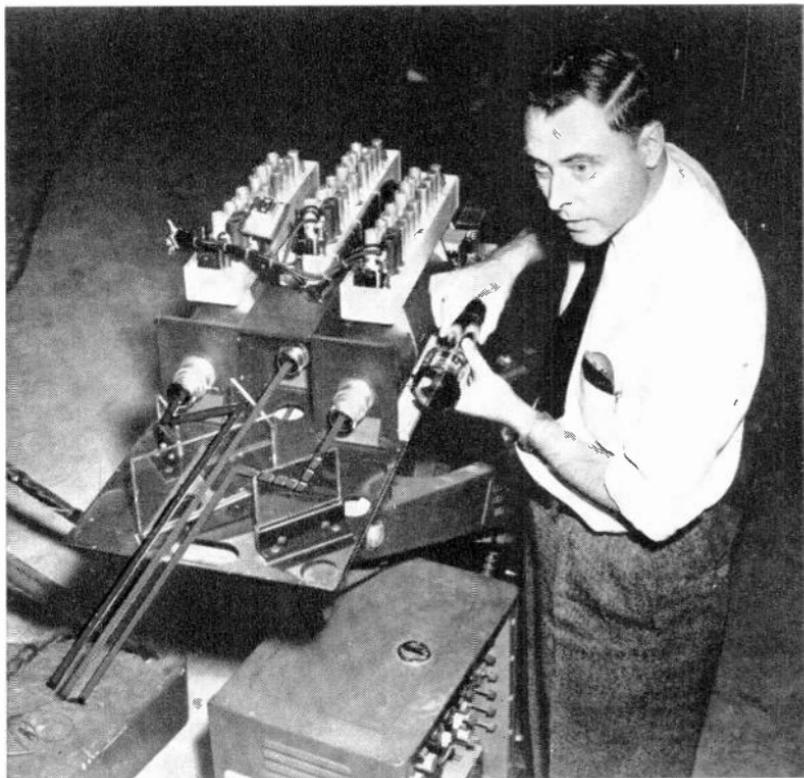
*Fig. 18-8.—The RCA color television camera with cover removed to show the system of dichroic mirrors and silvered reflectors which separate the color bands.*
