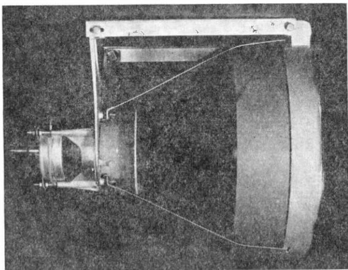
Fig. 10-1A. — A Du Mont 15-inch picture in its mounting.
