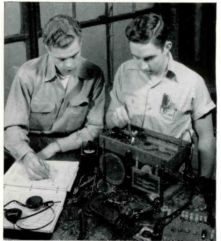
Coyne students testing specially built Power supplies. Some type of Power Supply is needed in every Radio or Television Receiver that uses Vacuum Tubes, so you see, the building of Receivers actually begins with the Power Supply.
