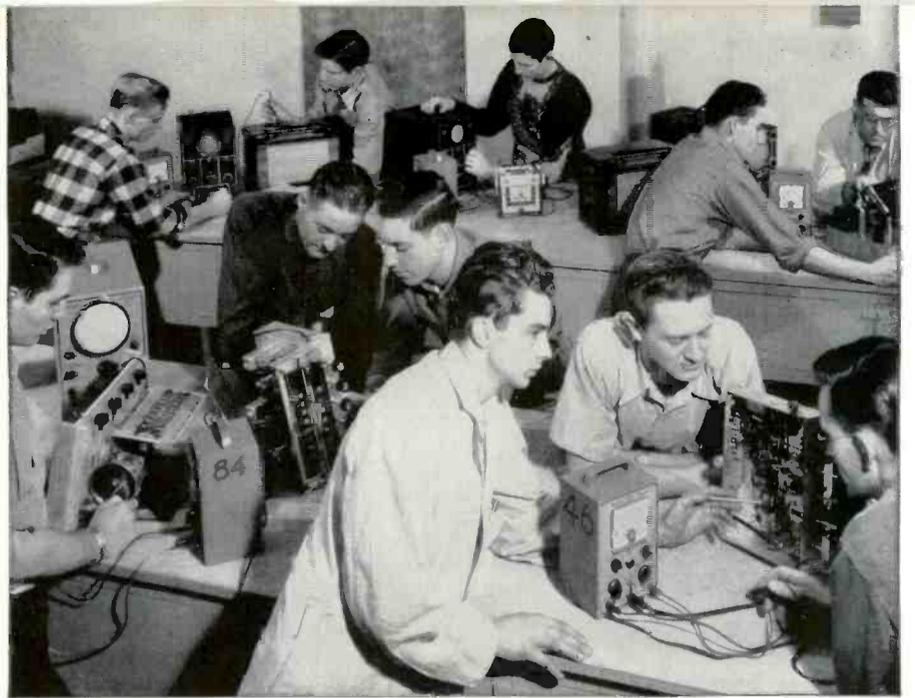
This photo shows you students using modern testing instruments to locate faults in various types of F.M. Tuners and Combination FM-AM Receivers. F.M. Circuits are used in all Television Receivers.
