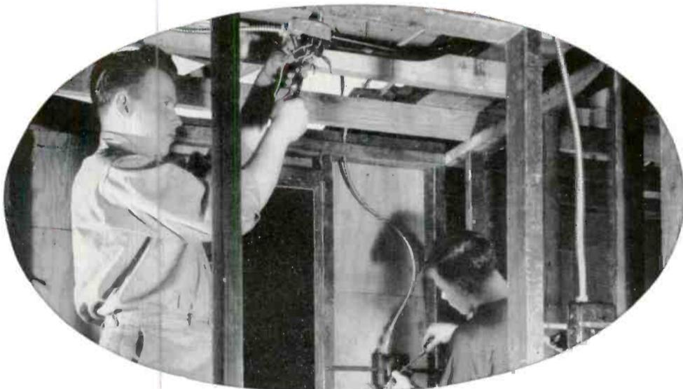
On certain house wiring jobs, the installation of BX, or armored cable is permitted in place of conduit.
