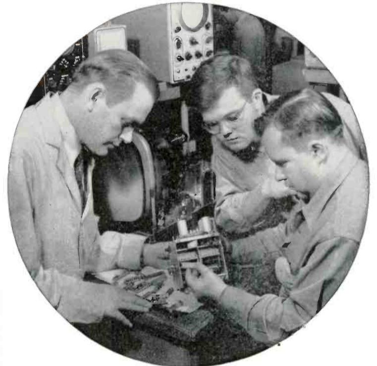
The photo above shows a section of our Television Service and Repair. This Coyne instructor is demonstrating the procedure of equipping a television receiving set to receive UHF (Ultra High Frequency) television.
