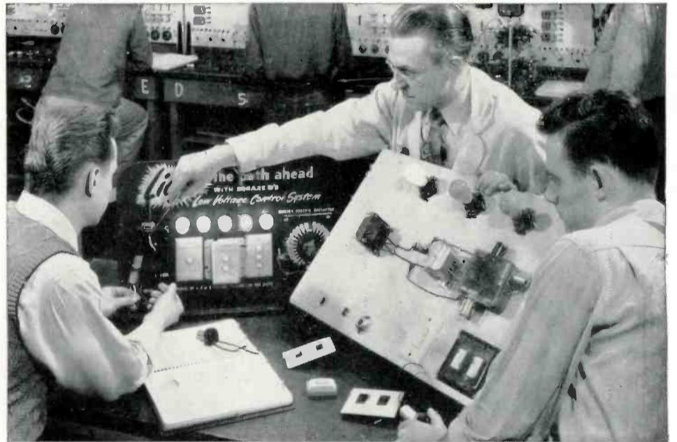
Here you see an instructor giving a demonstration on different makes of low voltage house wiring control systems. These controls are being used more and more in modern buildings.
