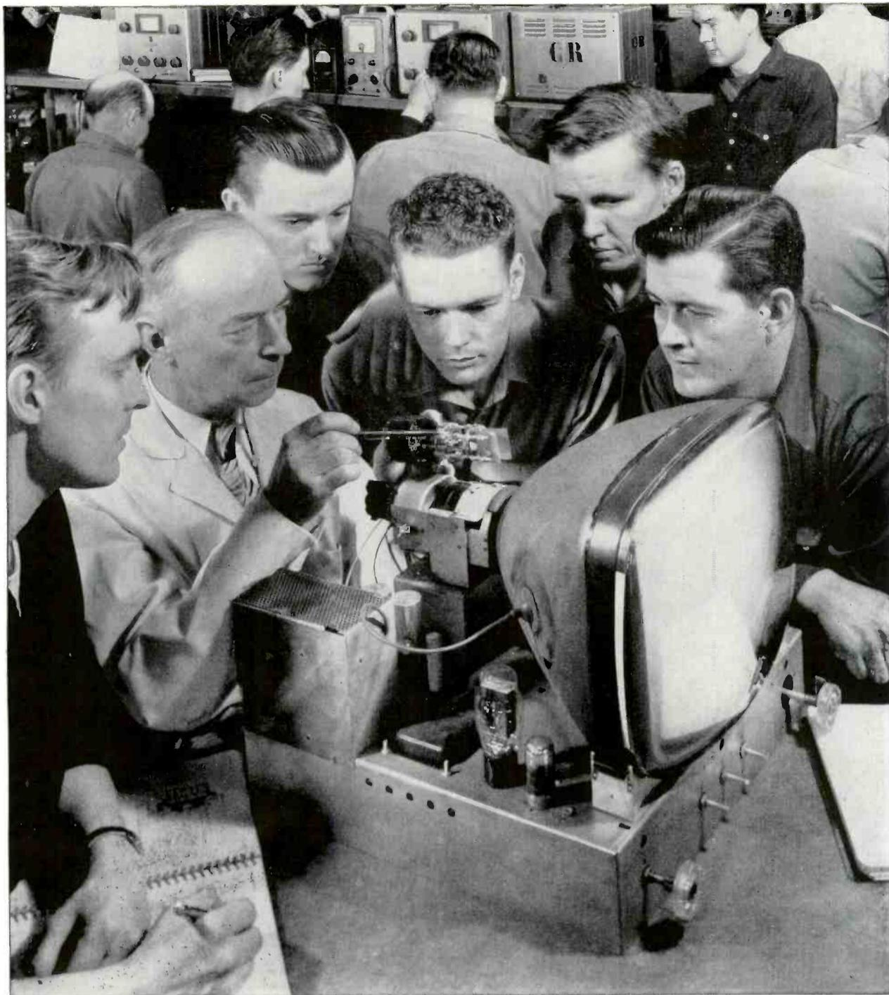
In the above photo we show an instructor giving a demonstration and explanation on how basic principles are utilized in the electron gun of a Television Picture Tube. The electron gun is the heart of a Cathode Ray Tube used in Television.
