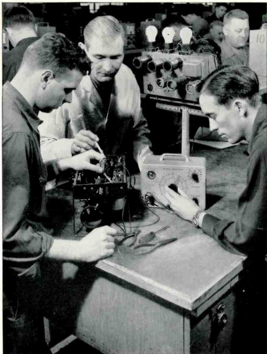
These students are building and testing Carrier Current Remote Control units, with which Electrical equipment, located some distance from the operator, may be turned off or on by means of high frequency impulses sent over Alternating Current power wires.
