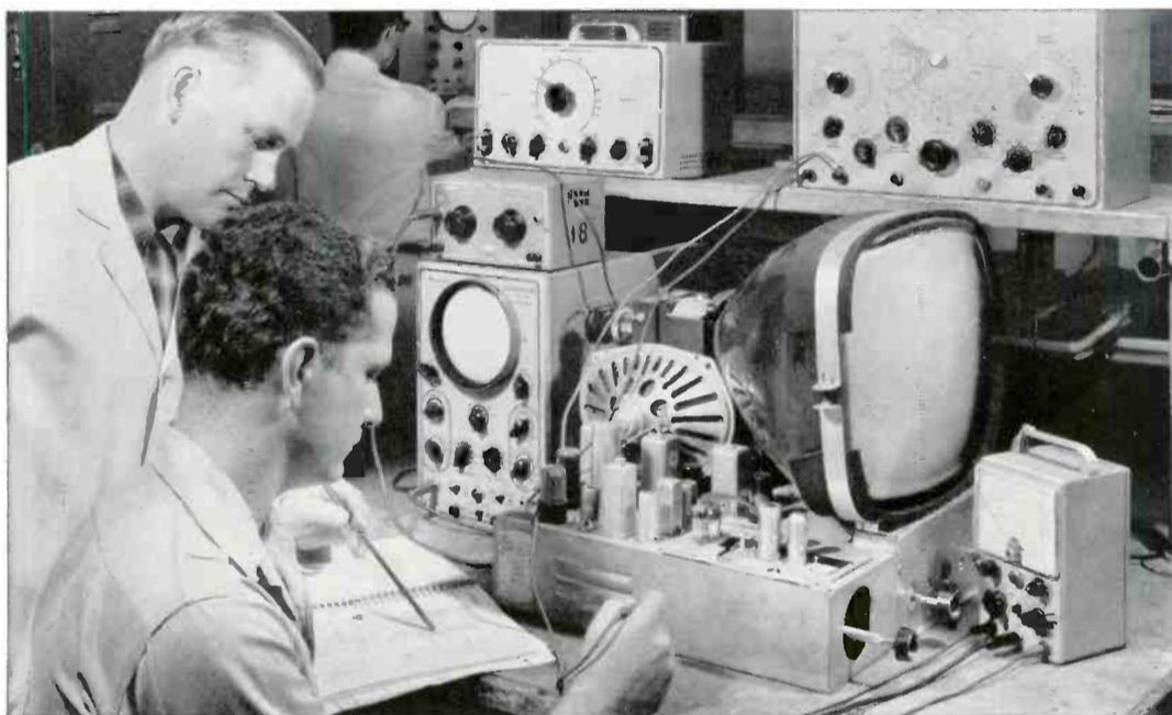
This student is getting special help from an instructor in measuring the strength of picture signals and checking for troubles that normally develop and making proper corrections to get the best reception.
