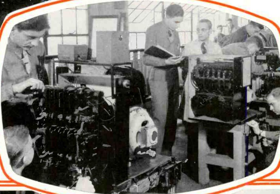
The photo to the left shows students learning care and adjustment of automatic and remote controlled A. C. motor starters, relays, contactors, coils and other equipment used in training students at Coyne.
