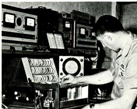
Besides Measuring Transmitter Frequency and Deviation, the Motorola Frequency Meter may be used as a Generator for "Netting" Receivers.
