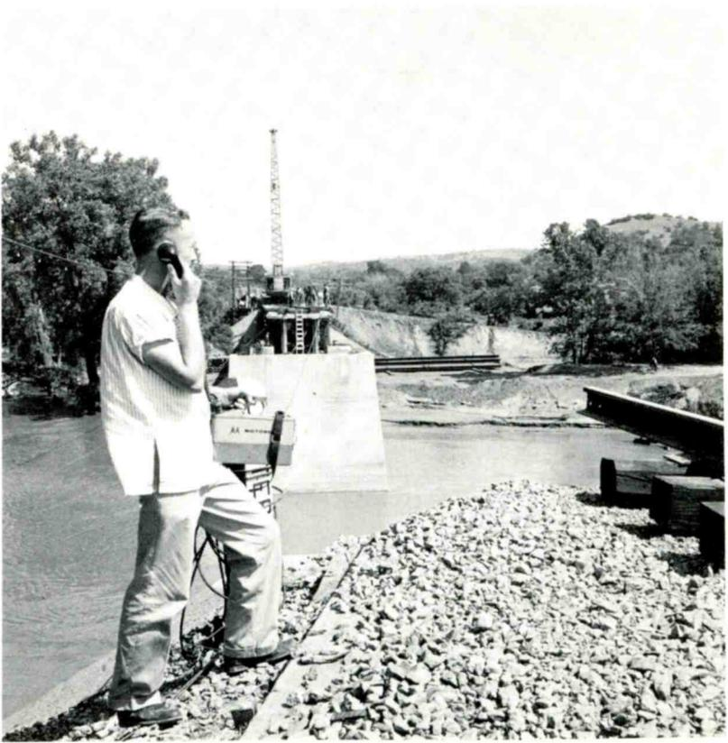
Construction foremen can communicate throughout project area when equipped with portable radiophones. Through extensive use of transistors such instruments are lightweight and low in power drain.
