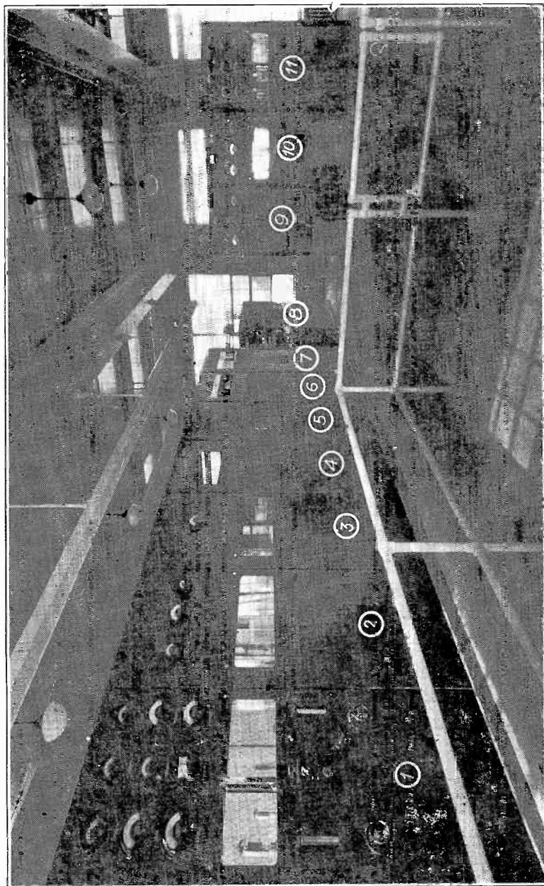
Western Electric 7-A 50 KW Transmitter. Units, left to right. (1) Crystal oscillator, crystal amplifier, buffer amplifier, modulated amplifier and modulator. (2) First power stage. (3) First power stage. (5) Final power stage. (6) (7) Tank circuit for final power stage. (8) Dummy antenna. (9) (10) (11) High voltage plate supply rectifier.
