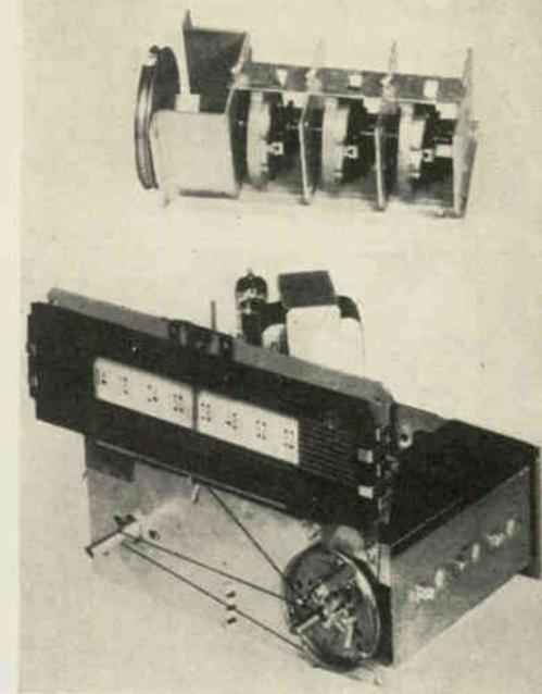
Fig. 1: (Above) Three section tuner used in P.R. Mallory's UHF-Converter (Below) converter and television receiver; 2. VHF—a-c power to television receiver on, VHF antenna directly connected to television input. Converter heaters on. 3. UHF—a-c power to both units and choice of separate UHF antenna, VHF antenna or built-in cabinet antenna depending upon signal conditions.
