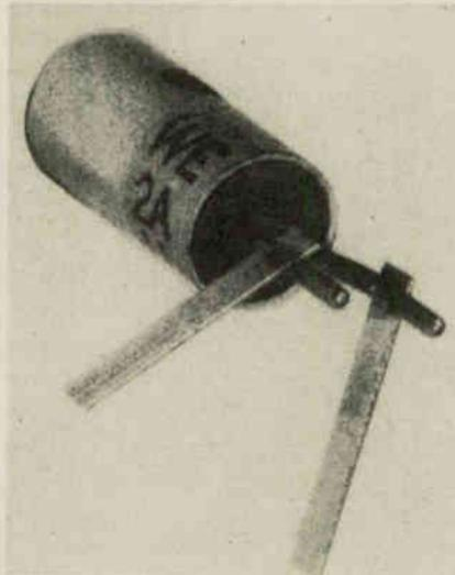
WESTERN ELECTRIC'S Type 2A transistor functions as an amplifier in the "card transistor" used with the new 4A toll crossbar system for automatic selection of routes in long distance telephone dialing. These units are used in conjunction with Type 3A phototransistors which are activated by light passing through a series of punched cards. The cartridge Type 2A has its base contact connected to the metal shell.
