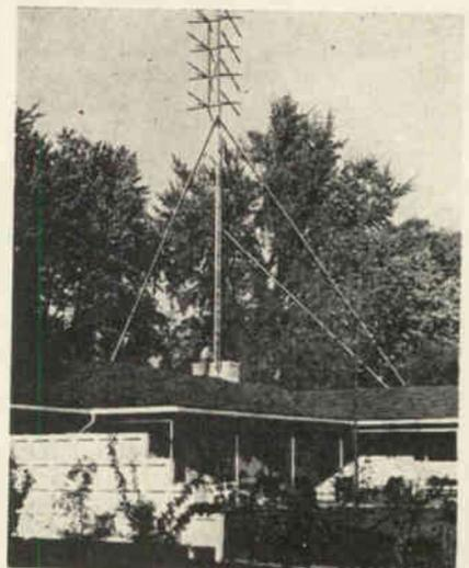
mount such antennas six or eight feet above the highest set of guy wires to permit a small amount of unrestrained motion. Many types of antennas make a roaring noise like that of an airplane under certain wind conditions. To avoid service callbacks, be sure to plug the top of the antenna mast with a large cork, and either place corks in the ends of the antenna elements or flatten them with pliers.
