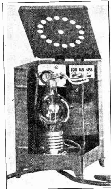
Fig. 30—General appearance of a commercial one tube rectifier with two sides and top removed.
