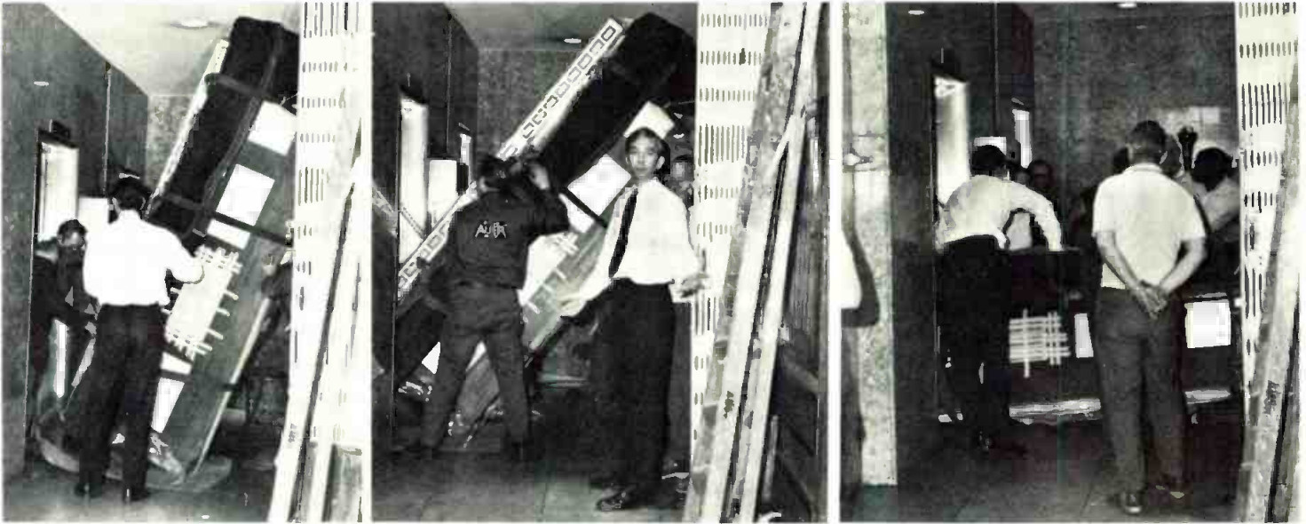
With blankets added the console is upended and brought to the elevator shaft where it is again placed horizontally.
