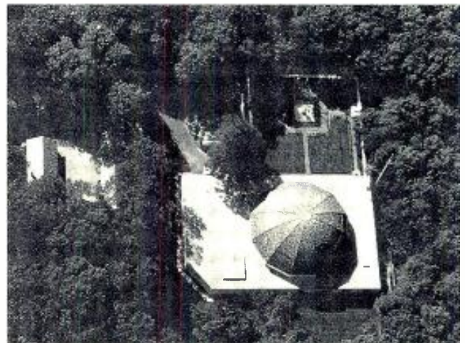
Figure 1. The Vanderbilt Planetarium. The domed portion is actually a separate building within the outer structure.
