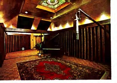
Golden Age Recorders in Culver City, California. This studio features a modular diffuser-slat design to optimize room ambience and increase reverberant field homogeneity. Bass absorption is accomplished by the ceiling resonator cove, and natural light provided by the four-paned acoustical skylight. Acoustic design by Jeff Cooper.
