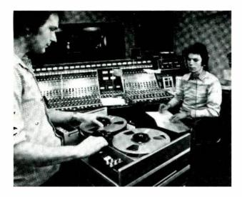
Figure 2. EMI Records audio engineers Colin Johnson (left) and Melvin Toms check out the prototype digital recording system prior to a recording session at Abbey Road Studio 3.
