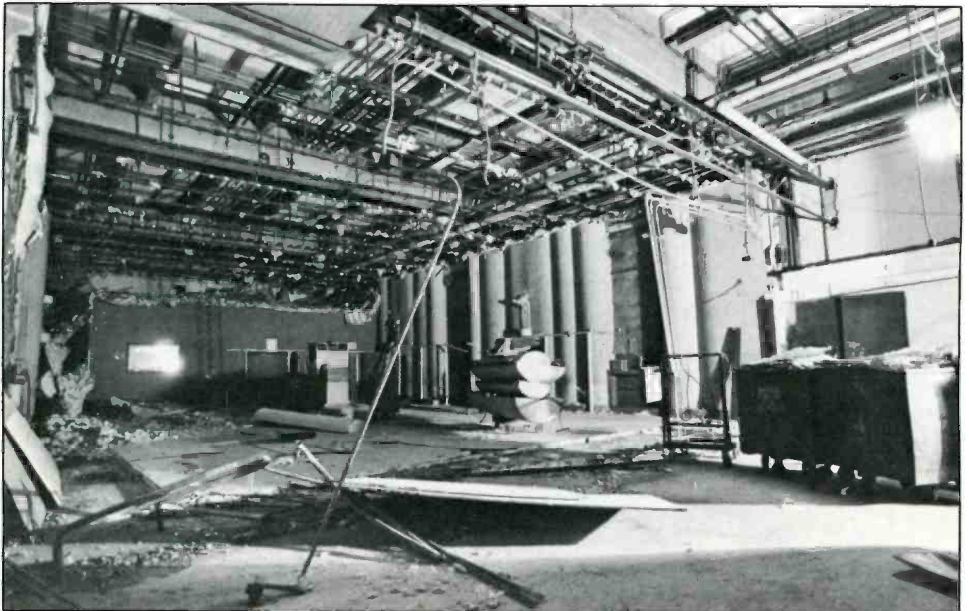
Studio under construction.
