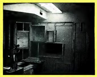
Wood formers before the walls are completed to allow placement of equipment.
