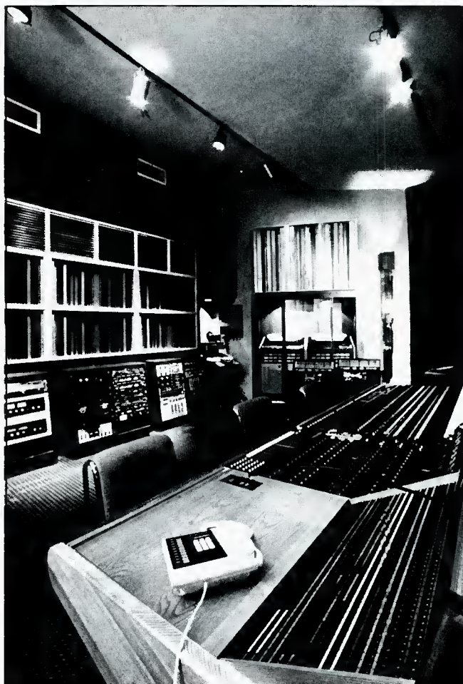
Figure 5B. Rear view of the control room at Master Sound Astoria in the Kaufman Astoria Film Studios, Astoria, NY, showing rear and side RPG diffusors. Acoustical consultant, Charles Bilello Associates.
