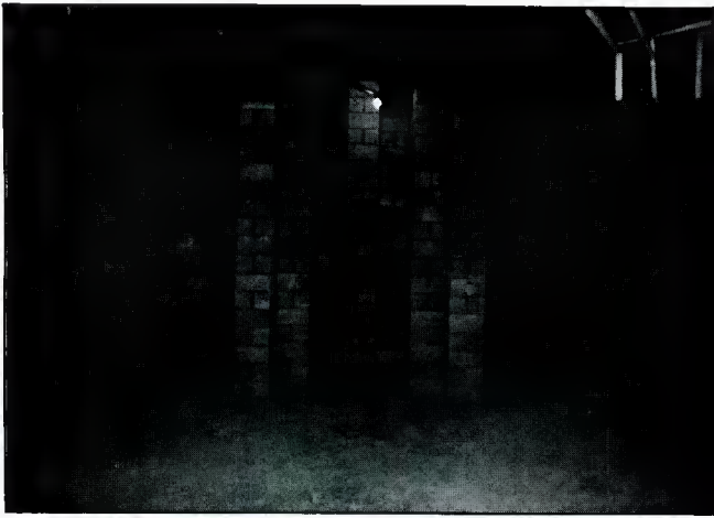
Figure 8A. Construction photo of cinder-block LFD.
