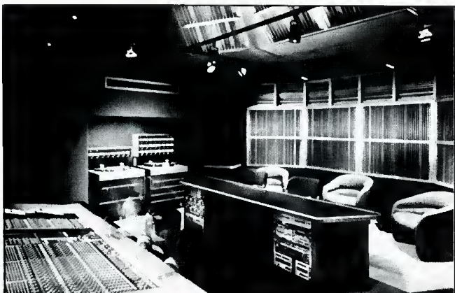
Figure 5A. Rear view of the control room at Tele-Image, Dallas, TX, showing upper and lower RPG clusters. Acoustical consultant Russell E. Berger-Joiner-Rose Group.
