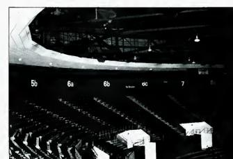
Figure 12. After acoustical modifications. Note the Helmholz cylinders.
