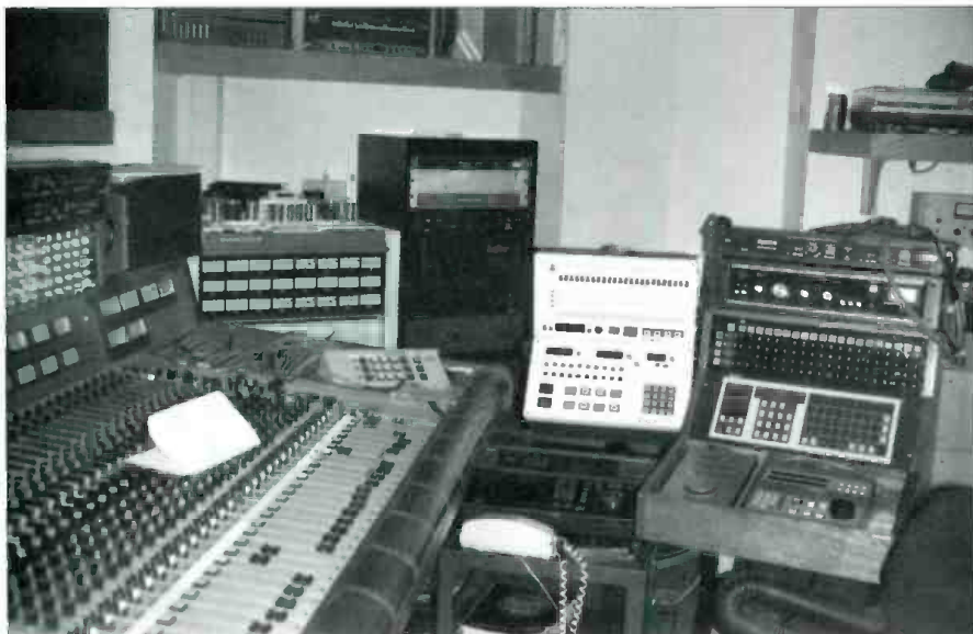
Figure 5. A completed studio 7 now ready for use.
