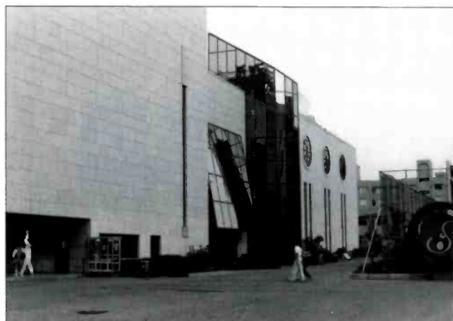
Figure 1. NBC's building at the International Broadcast Center in Seoul, Korea.
