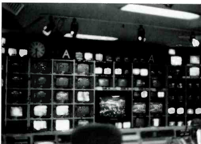
Figure 5. Control Room "A." The monitor wall gives an idea of the complexity of the coverage task.
