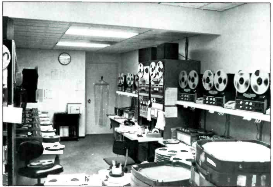
Figure 13. The tape duplication facility.
