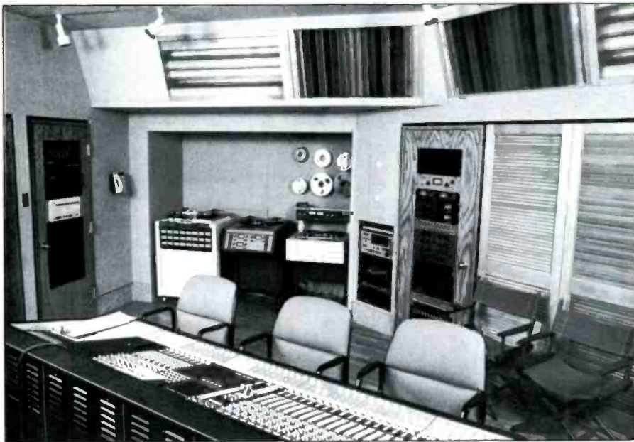
Figure 8. Studio 2 has an SSL 4000ETR and a 3-machine lock up.
