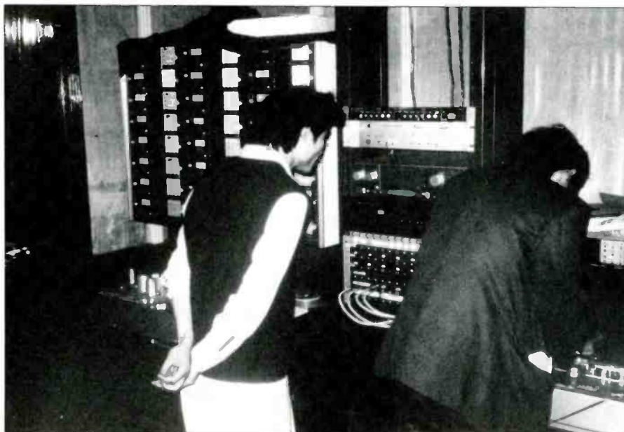
Figure 1. Making ready a master for playback in the tape machine room.
