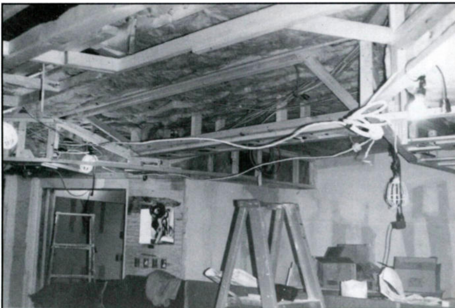
Figure 10. The acoustic ceiling nearly done.
